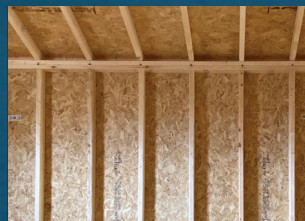
For Buildings with Painted LP Smart Panel Upgrade to 16" Trusses (Standards is 16" On-Center Studs and 24" On-Center Trusses)
