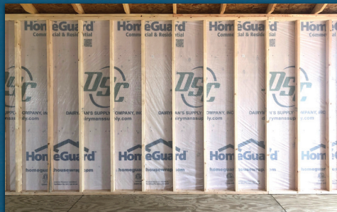
House Wrap Vapor Barrier Recommended if you plan to insulate
