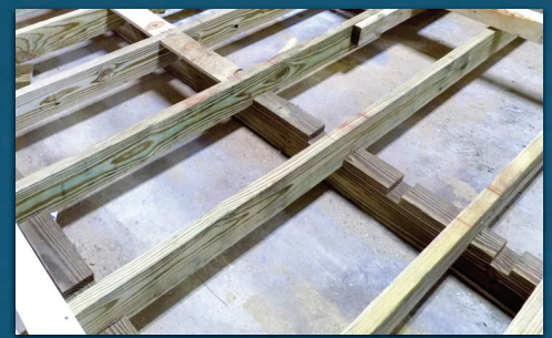
12" On-Center Floor Joists 16" OC is Standard
