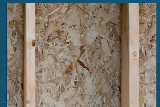
Upgrade to 2x6 Studs & Trusses
